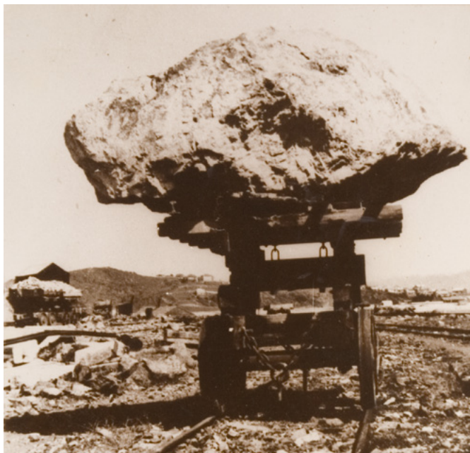
Construction of the breakwall, thought to have been taken in the late 1920's. (Courtesy of Coffs Harbour Museum)
