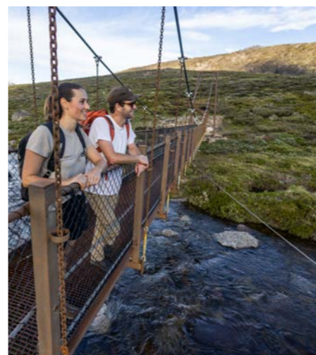
Spencers Creek bridge on the Guthega to Charlotte Pass walk. Photo: Boen Ferguson/DPE
